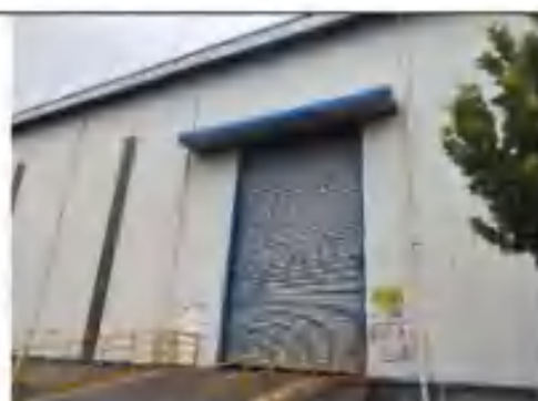
油泥砂贮存间北侧
